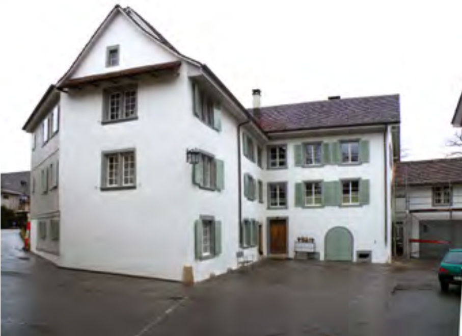
Figure 1: A historical demonstration building from the 15th century with a 6 cm of exterior aerogel render insulation
