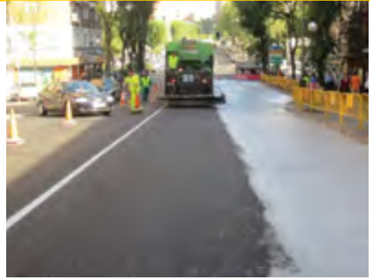
Figure 2. Slurry application in Madrid city center (2012)
