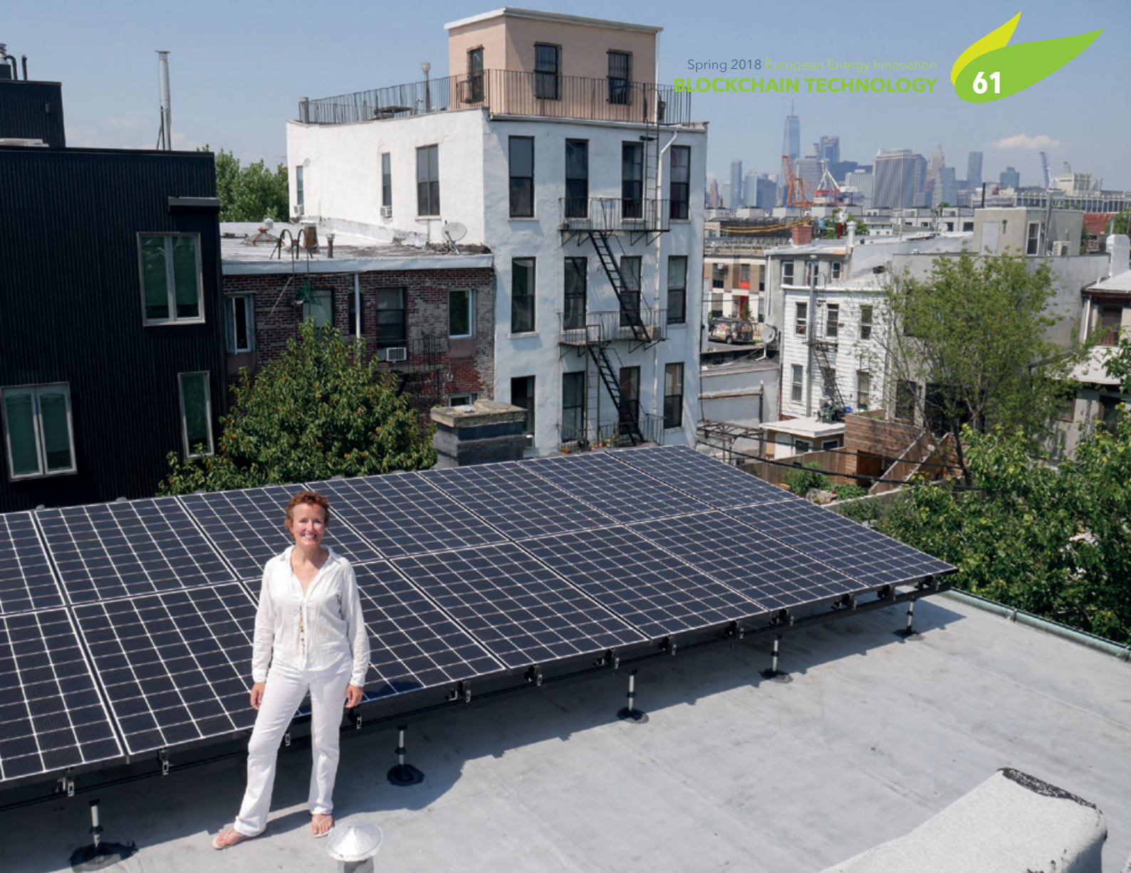
Victoria Milne, Brooklyn microgrid prosumer, on her rooftop with her solar PV system (Photo LO3)
