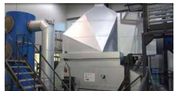
8 MW heating plant in Bogense, Denmark.
