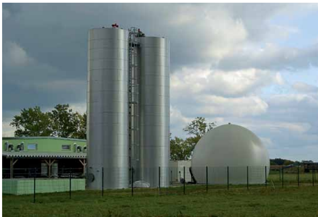
Top: wood pellets. Bellow: biogas plant
