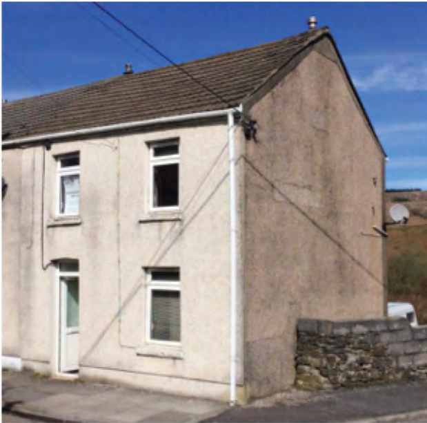
Picture of a before and after retrofit house
