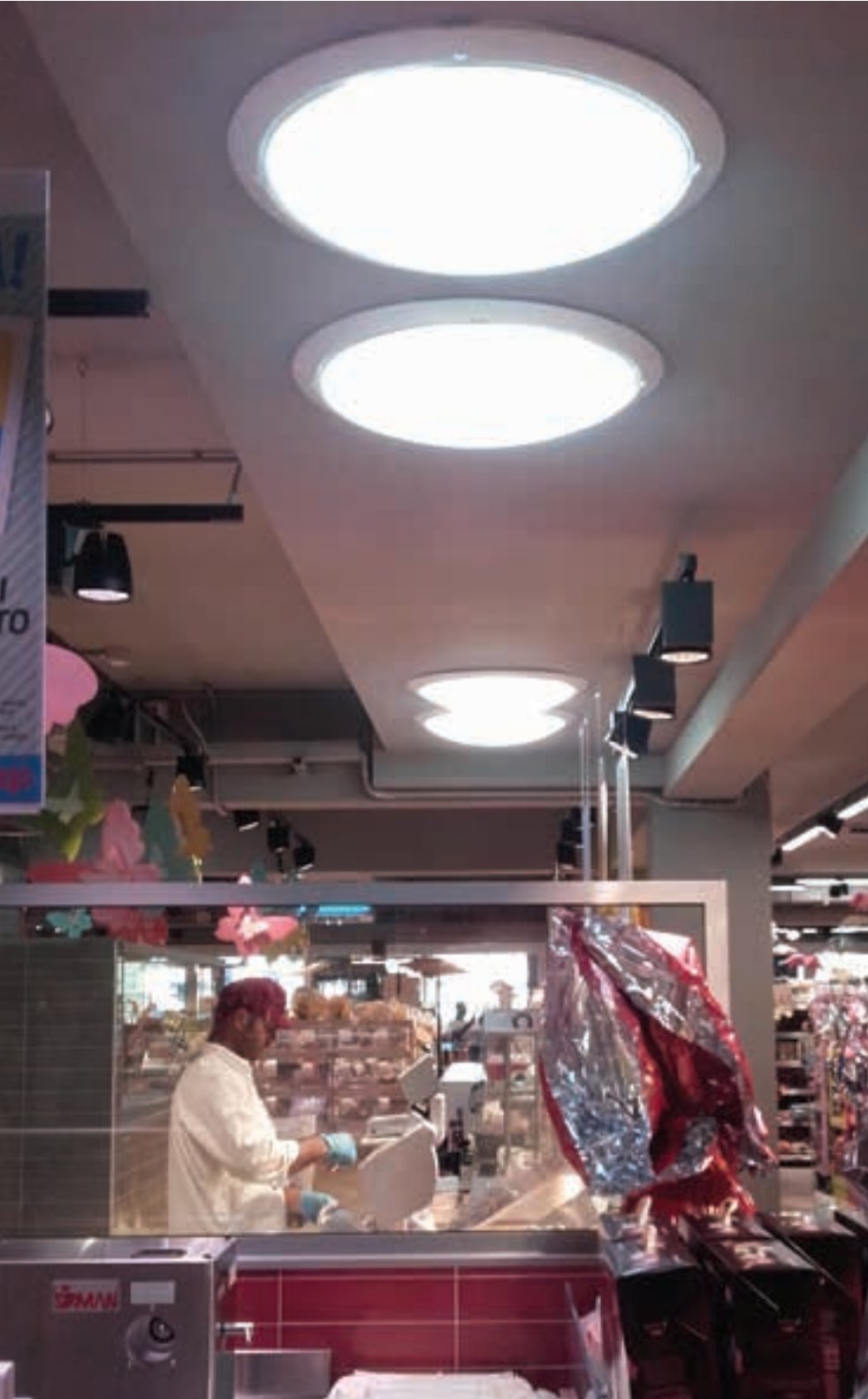
Figures 3 and 4 - Solar tubes in the shopping centre “Modena Canaletto”, bringing direct sunlight inside the shop. Source: CommONEnergy, http://commonenergyproject.eu/
