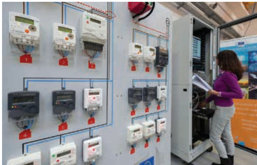
Smart Grids Interoperability Laboratories: The Smart Grids Interoperability Laboratories at JRC Ispra and Petten support the development of the EU policies by testing of the interoperability of the devices and systems that are part of the power grid.
