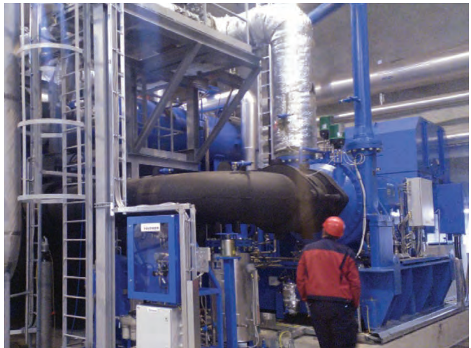
Large scale heatpump's from Friothersm to District heating purposes.
