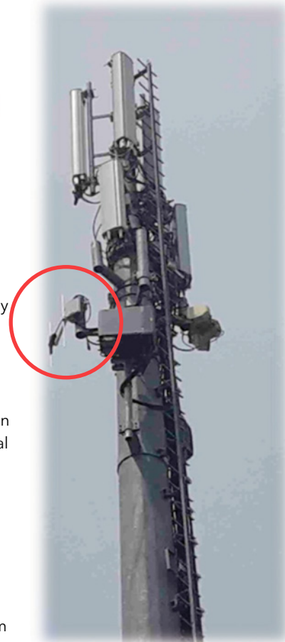
Capillary network concentrator/gateway on a Telecom Italia’s asset
